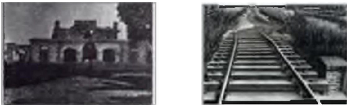
Figure 1.5: Damage of building in 1897 earthquake and damage of rail track in 1997 earthquake
