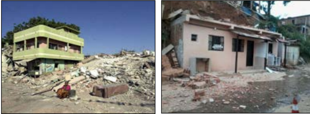
(b) RCC buildings (Bhuj Earthquakes 2001, India (Datta, 2001))
