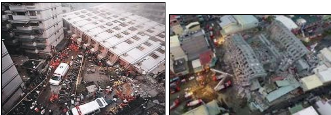
(b) RCC buildings (Taiwan earthquake, 2016 (NDTV, 2016))
