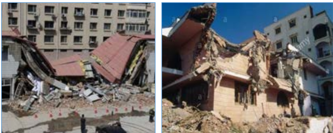
(a) URM buildings (Bhuj Earthquake 2001, India (Dinodia Photos RM, 2001))
