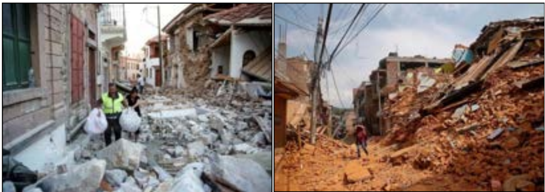
(a) URM buildings (Nepal earthquake, 2015 (Masood, 2015))
