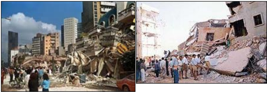
(a) URM buildings (Bhuj Earthquakes 2001, India (Singhania, 2016))
