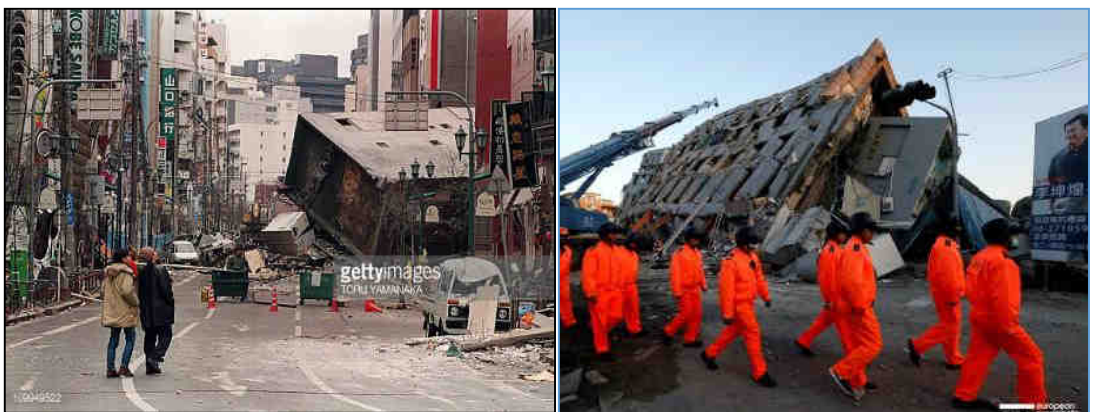
(b) RCC building first condition (Great Hanshin Earthquake 1995, Japan (Yamanaka, 1995))
