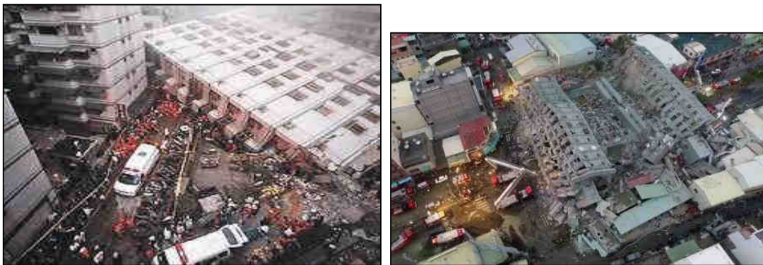
(b) RCC buildings (Taiwan earthquake, 2016 (NDTV, 2016))
