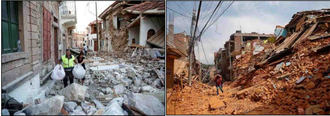
(a) URM buildings (Nepal earthquake, 2015 (Masood, 2015))
