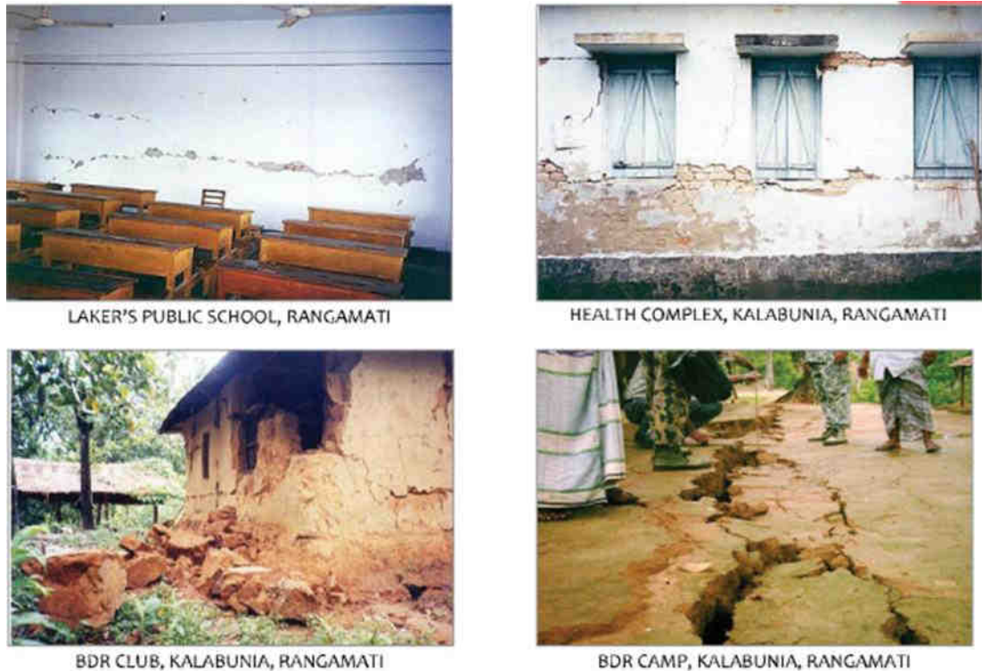
Figure 1.4: Damage of earthquake in Kolabunia, Rangamati after 2003 earthquake
