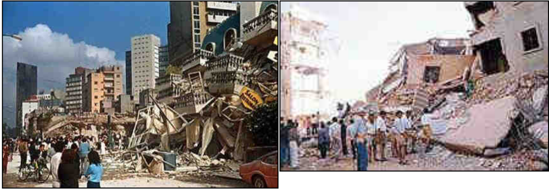
(a) URM buildings (Bhuj Earthquakes 2001, India (Singhania, 2016))
