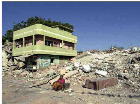
(b) RCC buildings (Bhuj Earthquakes 2001, India (Datta, 2001))
