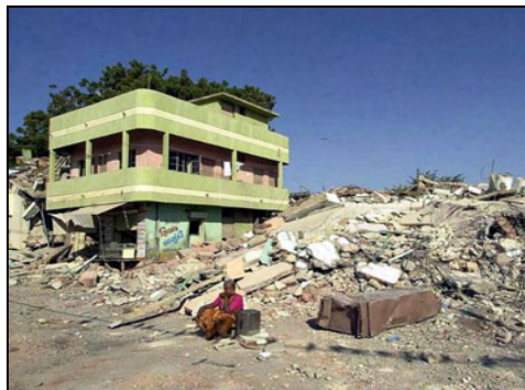
(b) RCC buildings (Bhuj Earthquakes 2001, India (Datta, 2001))
