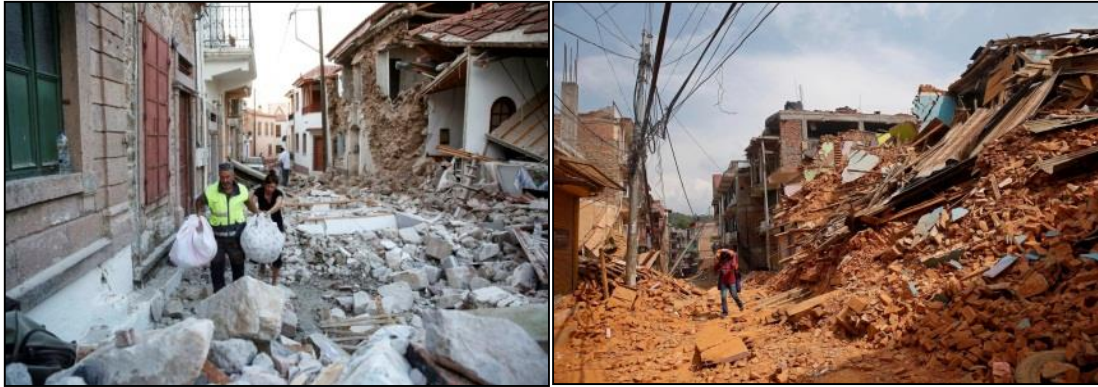
(a) URM buildings (Nepal earthquake, 2015 (Masood, 2015))
