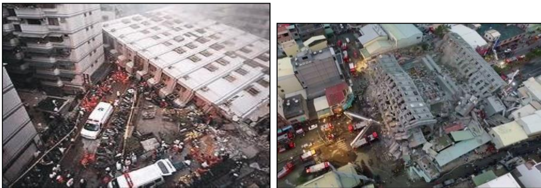
(b) RCC buildings (Taiwan earthquake, 2016 (NDTV, 2016))
