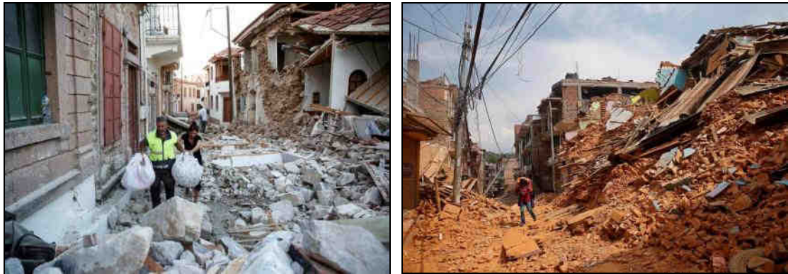
(a) URM buildings (Nepal earthquake, 2015 (Masood, 2015))
